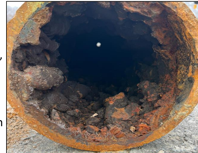
Route 46 – Transmission Main Replacement
