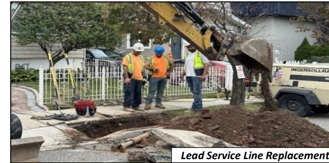
Lead Service Line Replacement
