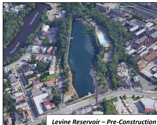
Levine Reservoir – Pre-Construction
