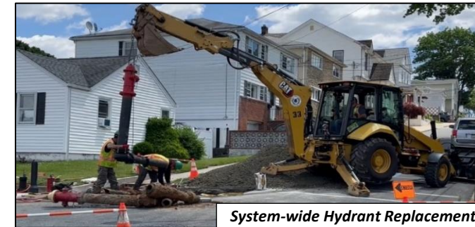
System-wide Hydrant Replacement
